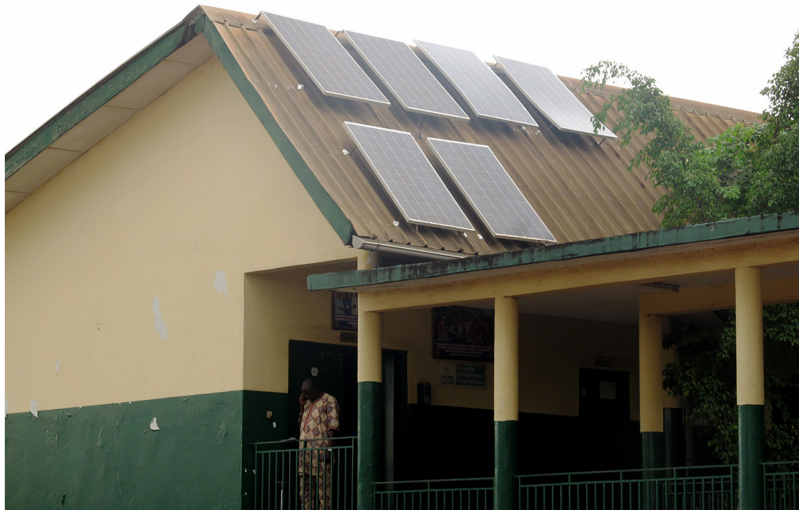
APC provided six solar panels to Flamboyants CHC. The electricity generated by the solar panels powers the water pump and the slit lamp in the ophthalmology ward.
